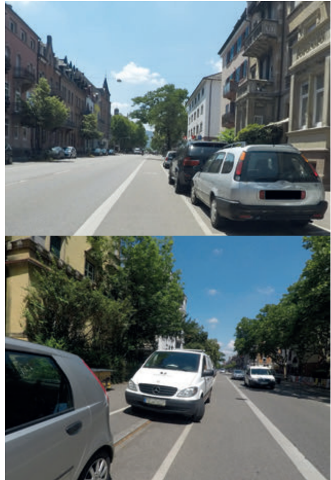
Figure 7: The absence of a safety strip may make dooring accidents more likely
