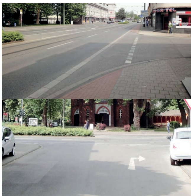
Figure 16: Unmarked (undetectable for vehicle drivers turning into and off the main road) cycle path priority (different views)
