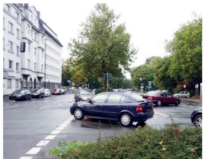
Figure 11: Impaired view for traffic turning left due to planted center strip and vehicles traveling in the opposite direction
