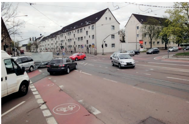
Figure 13: Worn-away/absent guidance and wait lines in junction (accident chart Figure 12)
